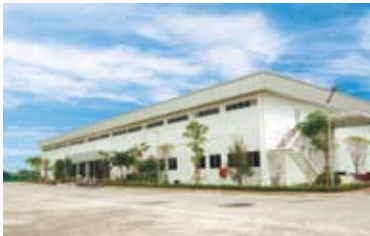
Energy-saving plant built in Bang Pa-in Plant, Thailand
