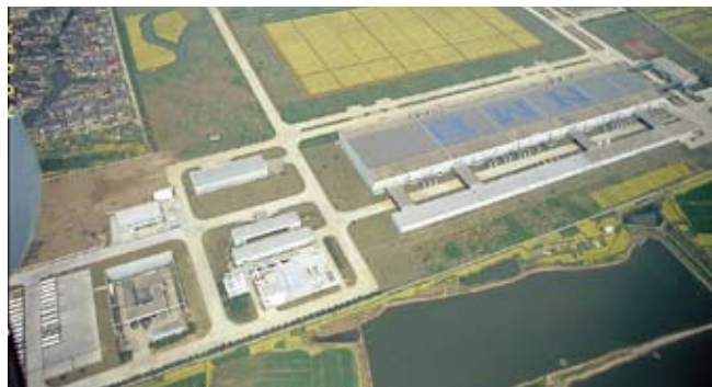
The Minebea plant in Shanghai, China, which has achieved zero output of industrial effluent
