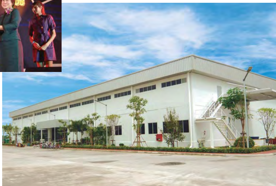
Energy-saving plant built in Bang Pa-in Plant, Thailand
