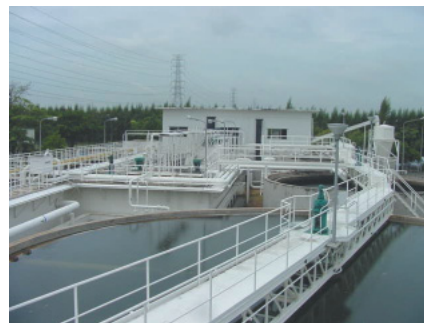
Wastewater processing facilities (Bang Pa-in Plant)
