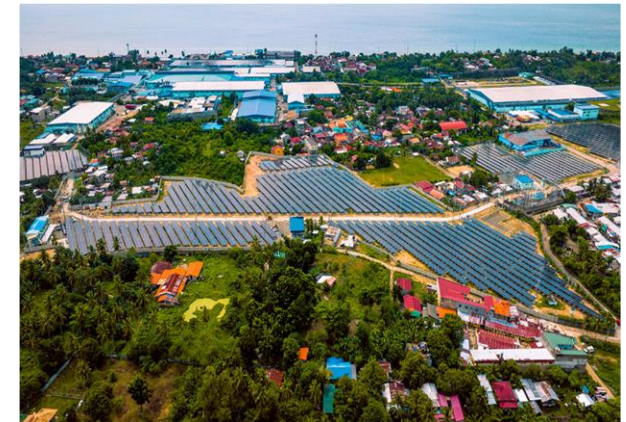
Solar panels installed at Cebu plant
