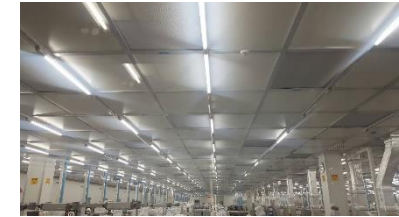
LED lights Installation at plants.
